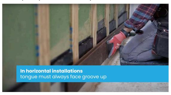
Use furring strips 1" x 2" (per local codes), maximum 16" apart, on top of sheathing\* and house wrap. In horizontal installations, tongue must always face up
