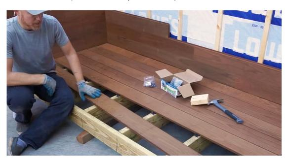
▶ Minimum gap between boards: 3/16". Mantis®, TurboClip®, or Invisi-Fast® systems automatically space the boards. Clips must be matched to the groove that is milled.
